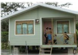
A house built with support from Fuprovi, in Costa Rica. Families contribute approximately 40% of the cost of the house with their labour.
